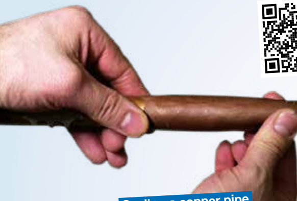
Sealing a copper pipe with Repair Stick Copper
